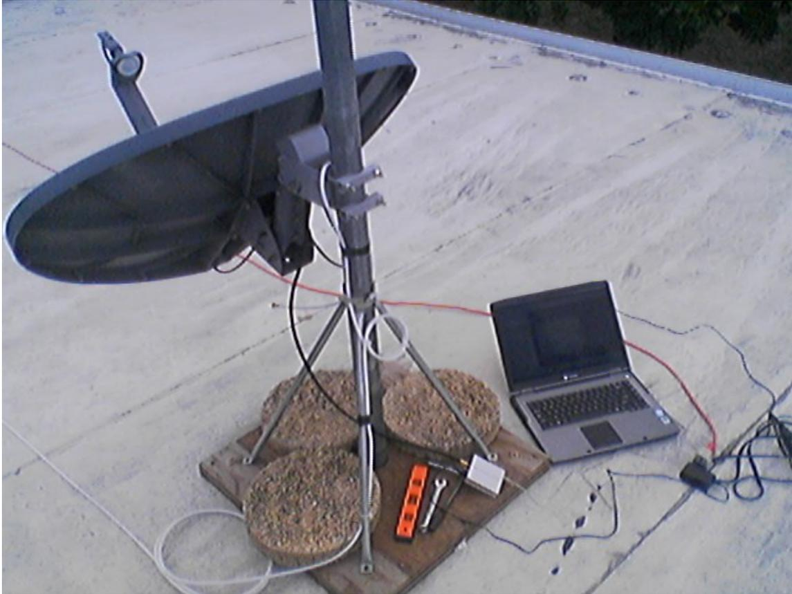
Fine tuning the dish is much easier with the QQ Box. Display the channels signal quality from DVB Dream “Scan Transponder” window.
