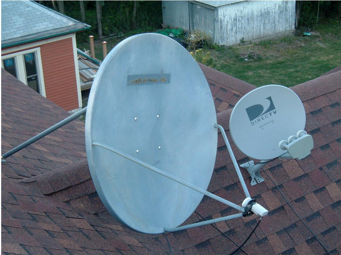
I have GREAT results on getting Ku transponders on these dish!!! Most of the LNBF necks fit into the LNBF holder. Remember, if these dish are on a motorized system, you do not have to skew the LNBF. Otherwise, it must be skewed as well as the dish has to be set with elevation, etc (fixed Satellite dish).
